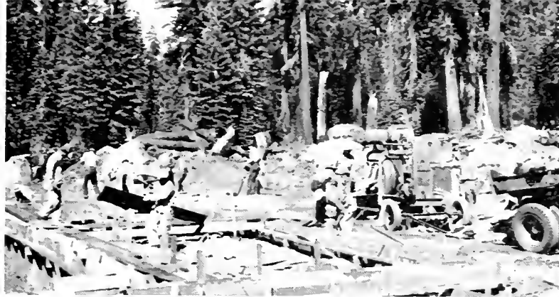
Pouring concrete on bunkhouse foundations, Sept. 23
